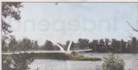
Rosales and Partners — Schlaich Bergemann and Partner Joint Venture Et Al., created this breezy design.
