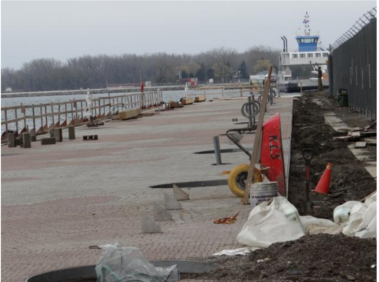
Portland Slip Project Construction, image by drum118
