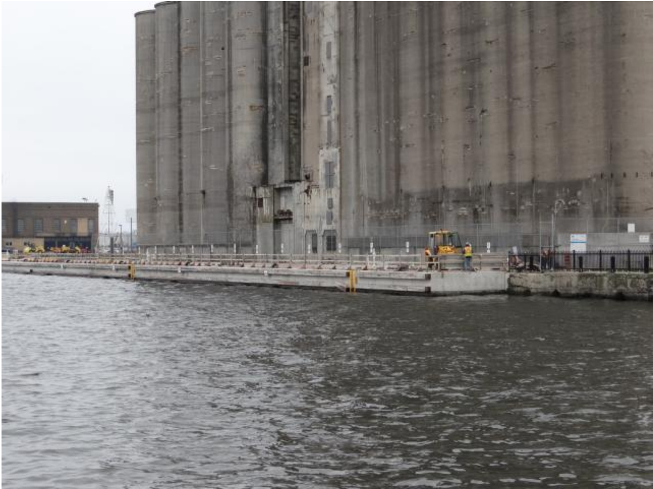
Portland Slip Project Construction, image by drum118
