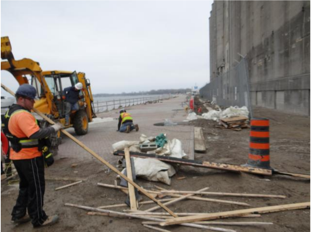
Portland Slip Project Construction, image by drum118
