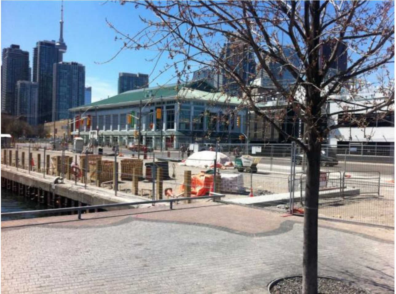
Central Waterfront Promenade Construction against Queens Quay, image by canadain
