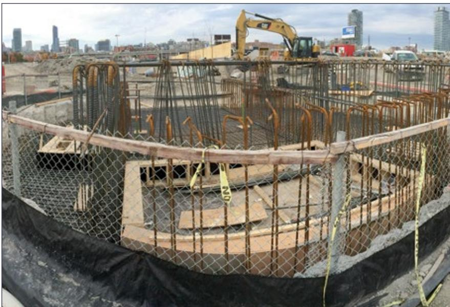
Stormwater attenuation shaft roof slab and access chambers under construction (October 2014).
