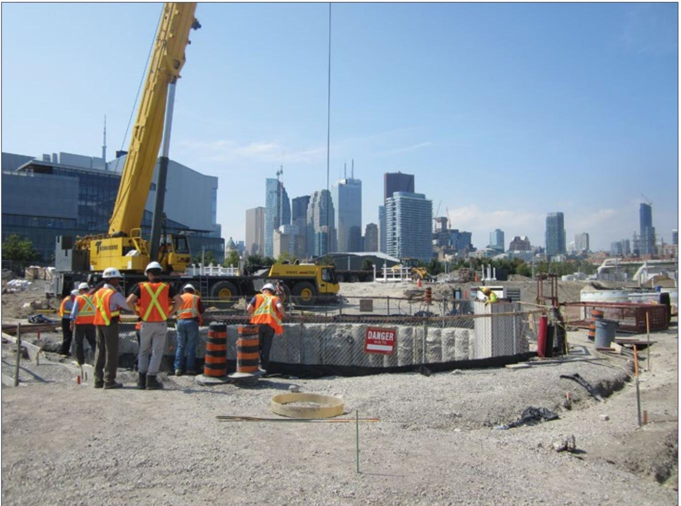
Vertical walls of the stormwater attenuation shaft under construction (August 2014).
