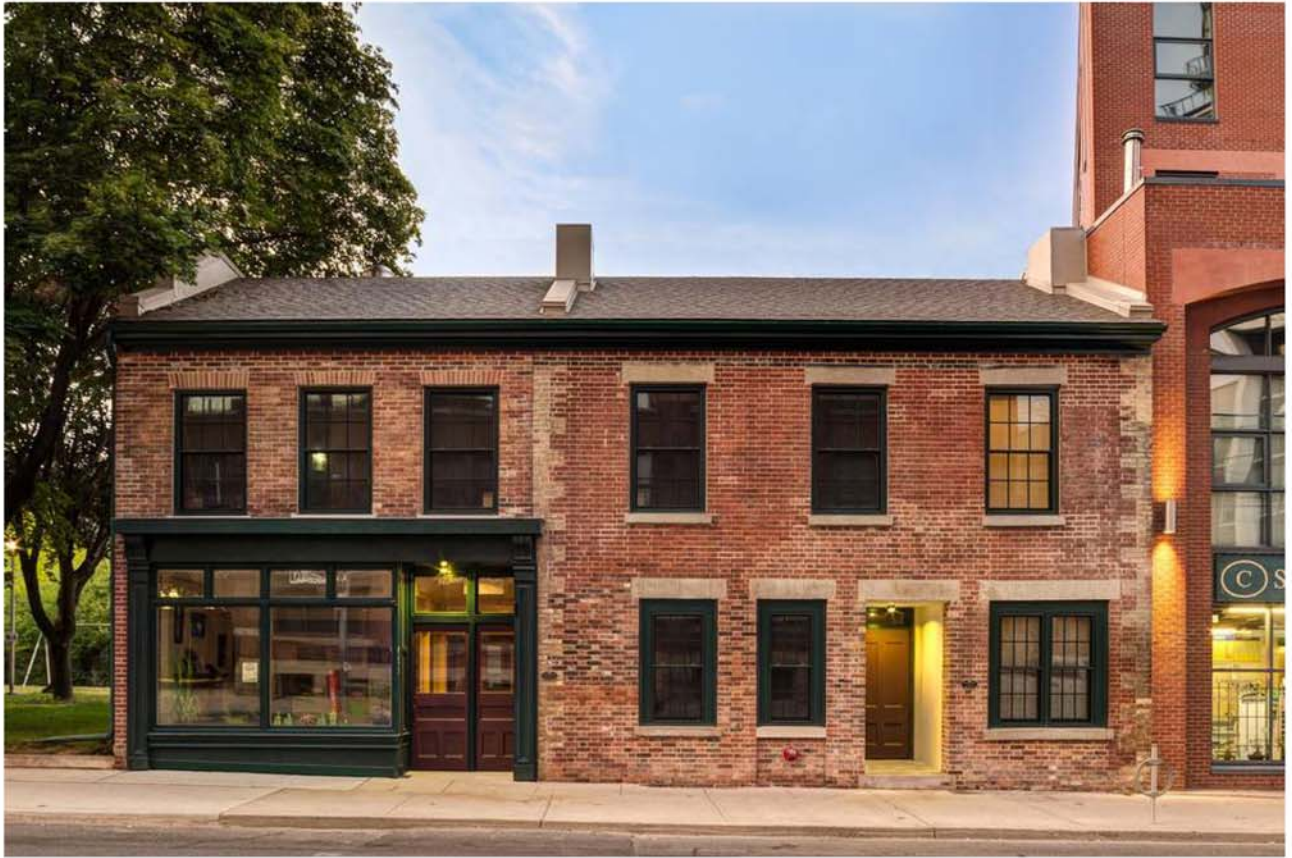
The Francis Beale Buildings, after restoration by DTAH. (Photo by Amaud Marthouret)
