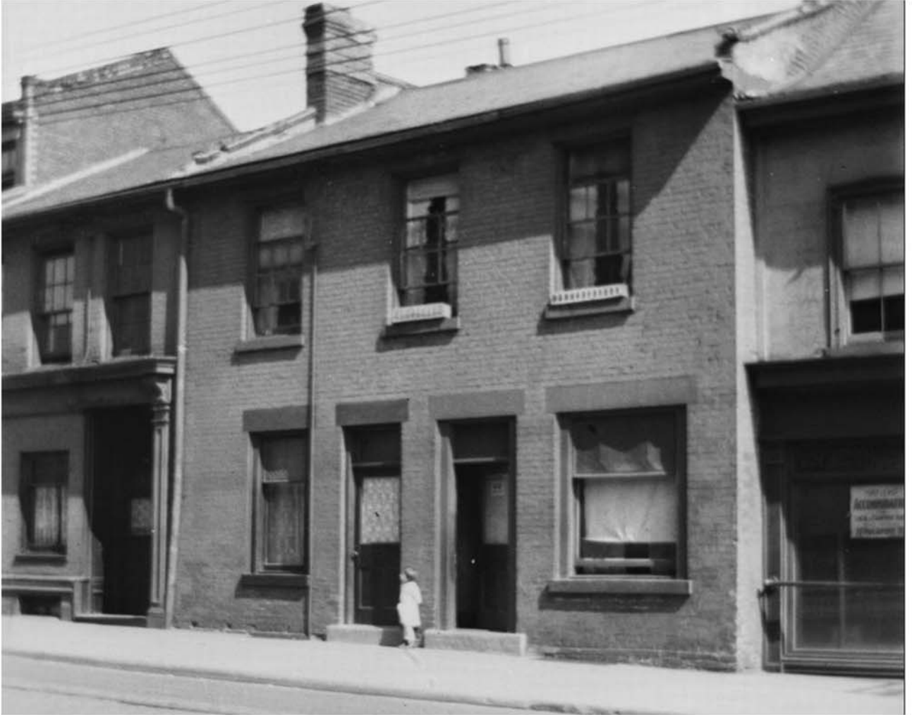
The pre-Confederation Francis Beale Buildings, 399-403 King St. E., circa 1930, left, and the condition before restoration work began.
